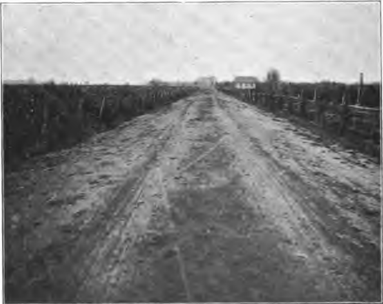
Elmer and Alloway road, Salem Co., after improvement.
